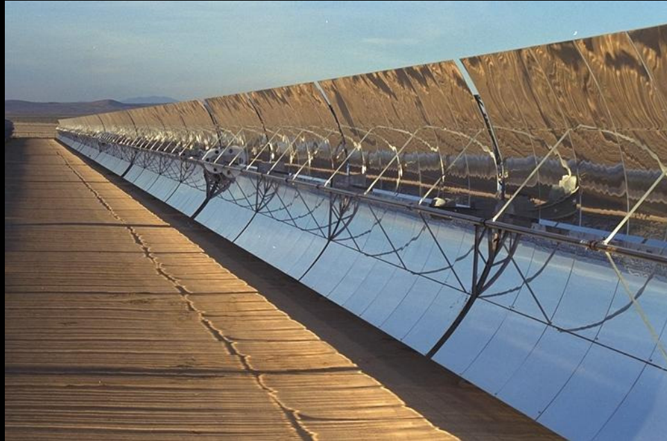
Parabolic Troughs (Concentration Ratio \sim 80 )
