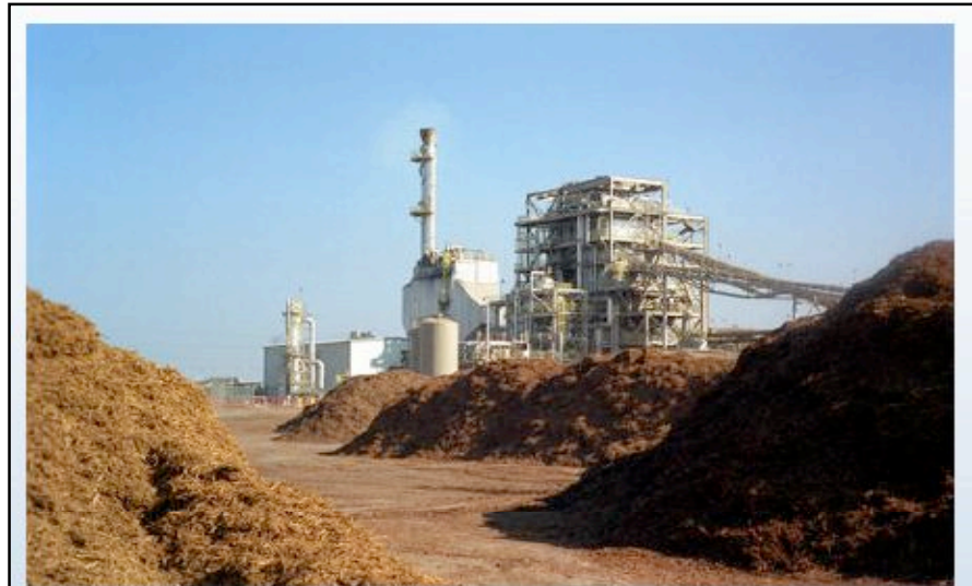
Rated at 21 MW and providing the San Francisco Bay Area with baseload capacity, the Tracy Biomass Plant uses wood residues discarded from agricultural and industrial operations.
