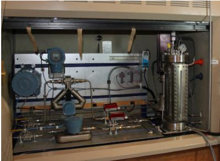
Fuel mixing system
