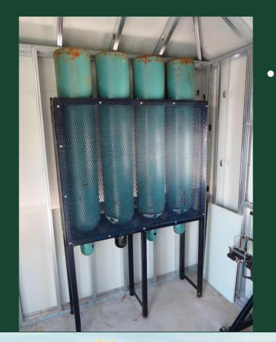
The ammonia vapors and residual gases flow into the outlet cylinders where the NH3 condenses and flows into a collector tank that is near the floor.
