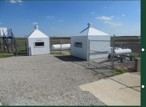
1000 gallon nitrogen storage tank is behind shed, and mobile NH3 storage tank is on near side
